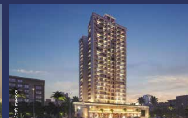
SAI AARADHYA KHARGHAR G+22 Storeyed Tower
