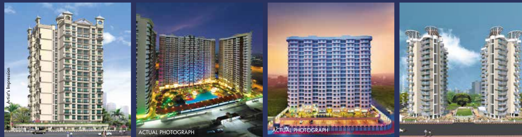
ACTUAL PHOTOGRAPH ACTUAL PHOTOGRAPH ACTUAL PHOTOGRAPH ARTIST'S IMPRESSION SAI JEWEL KHARGHAR G+18 Storeyed Tower SAI MANNAT KHARGHAR G+26 Storeyed Tower SAI RIVERDALE TALOJA G+19 Storeyed Tower with 2 Wings SAI PEARLS KHARGHAR G+15 Storeyed 2 Towers
